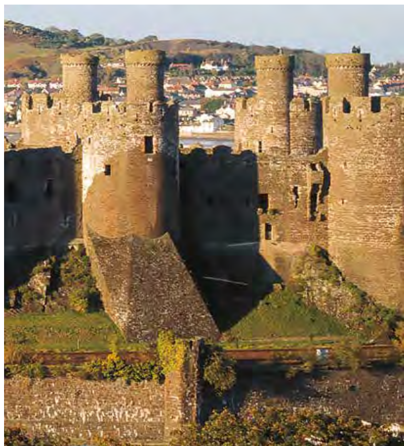
The repair to the Bakehouse Tower in Conwy Castle, made by the London and North Western Railway Company, is clearly visible as different coloured stonework in the middle tower.
