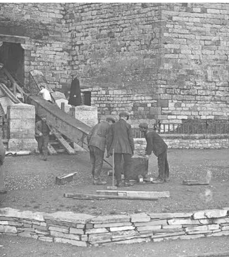
Restoration work at Caernarfon at the beginning of the twentieth century. Here, a massive oak beam is being brought into the castle from the quay echoing centuries of building practice.
