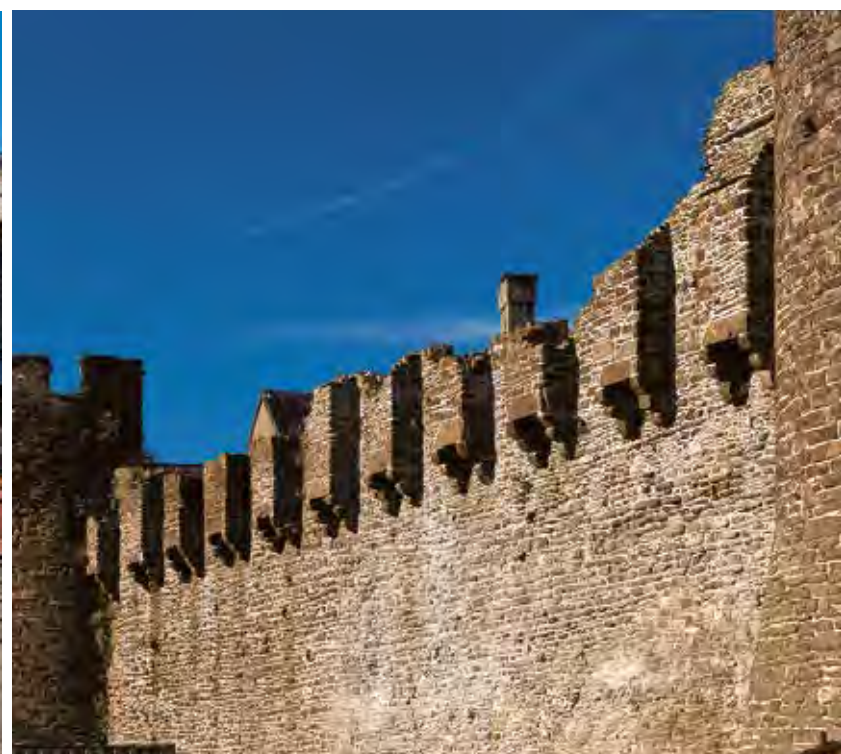
Medieval latrines projecting out over the town wall probably served the offices of medieval administrators located in a building on a site close to Rosehill Street.
